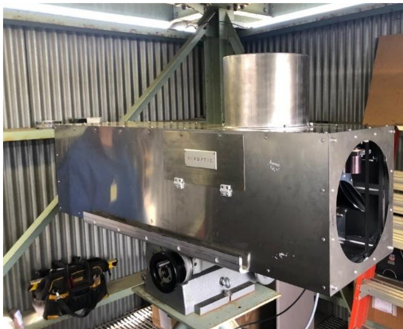
Airoptic TDL Base Unit Installed on Mounting Platform
